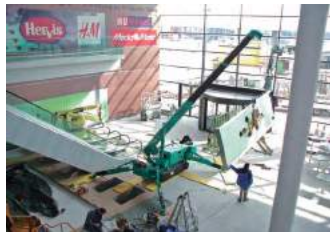
MC305C Panel Installation Mall
