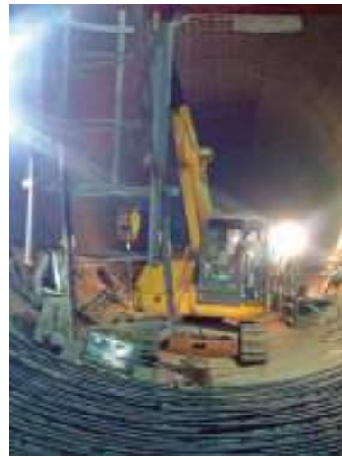
LC785 Flood Control Japan
