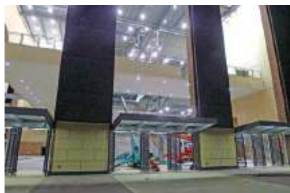
MC405C Sign Install - Inside Football Stadium US
