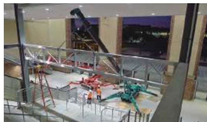
MC405C Steel Erection Kyle Field
