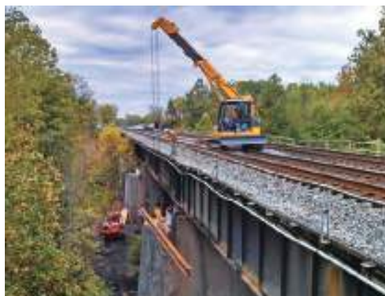
LC785 US Railroad Bridge - Active Track On Far Side
