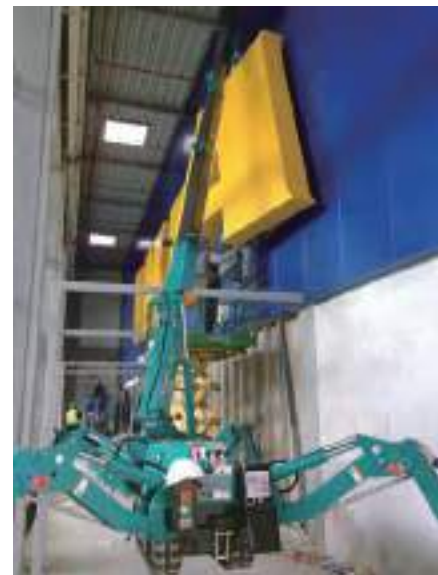
MC285C Sign Installation
