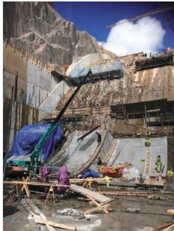
MC405C Power Plant Sweden
