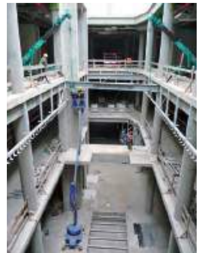
MC285C Construction Sky Tower
