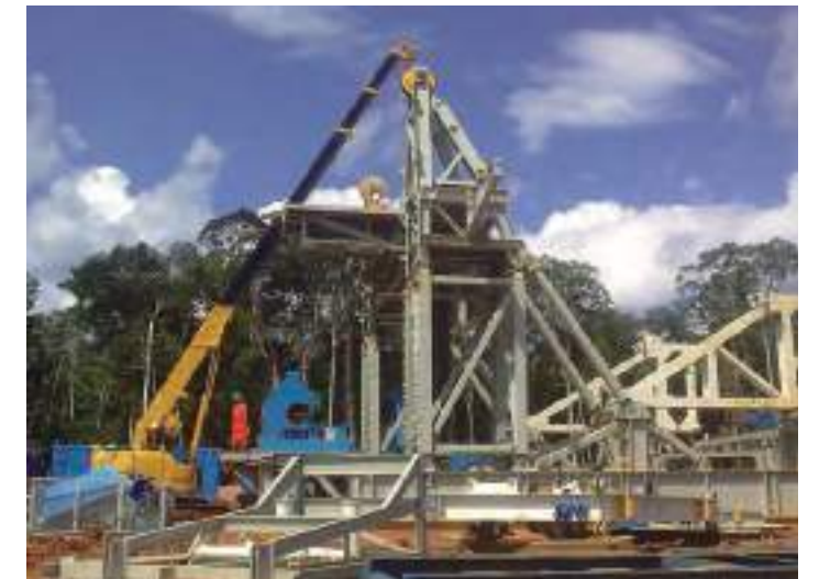
LC1385 On Site Rig Up of QG 5 Brazil
