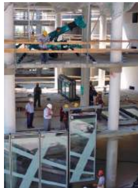
MC285C Construction Glass Lifting Bucharest
