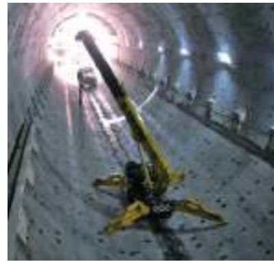
MC405C Tunnel Australia
